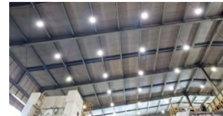
Replacement of lighting with LED fixtures
